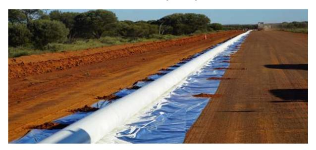
Through LPL, we are now once again driving the change from metals to composites, but this time the change is even greater, and we are the owner of the technology. LPL is delivering to the market the Fluid Highway®, which is a high performance, high pressure, composite alternative to the traditional fiberglass, steel and HDPE pipe.
